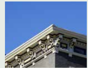
The cornice line of 116 W 14th Street is made up of decorative metal brackets and wood trim work
